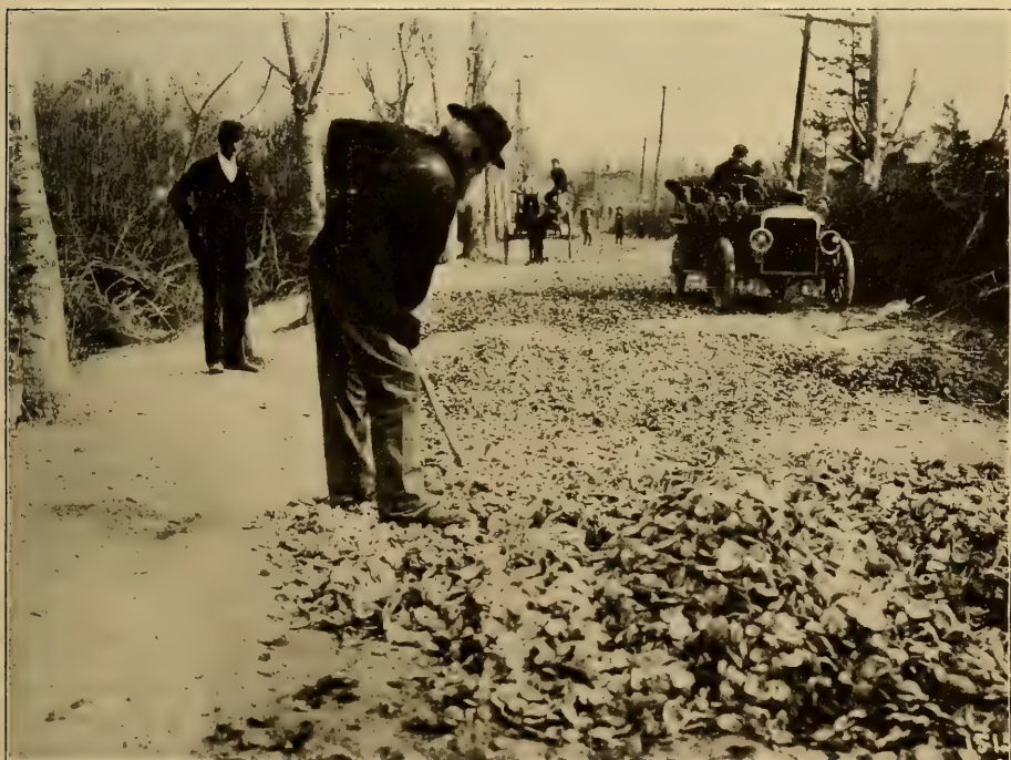
A shell road in the making—it pays to wait for the finished product.
